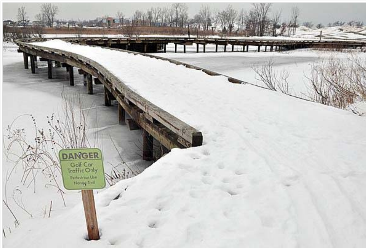
The cart path bridge leads to the seventh tee at The Golf Club at Harbor Shores, one of three holes built at Jean Klock Park in Benton Harbor. John Madill / H-P staff
